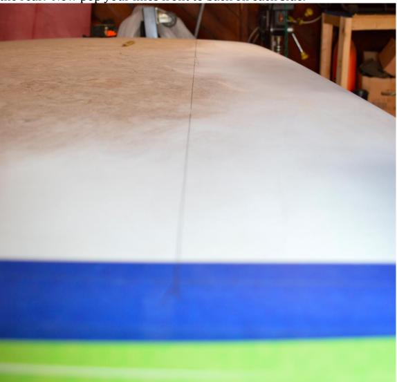
6. Make sure your marked hole lines are true. Make sure your width is the same through out from front to rear of the hole to be cut out and make sure your length is the same through out.
